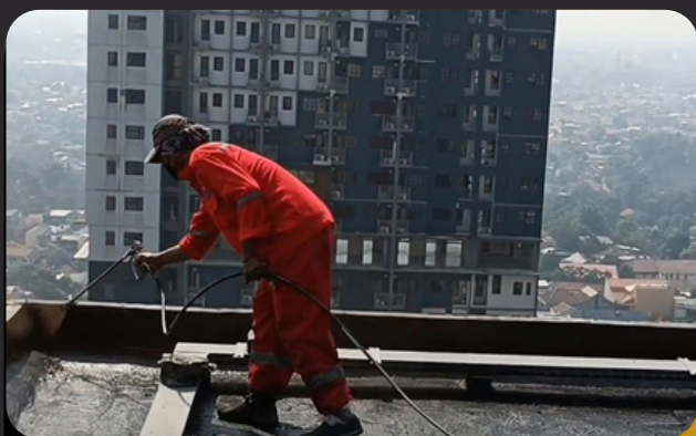
Waterproofing Dak Beton
